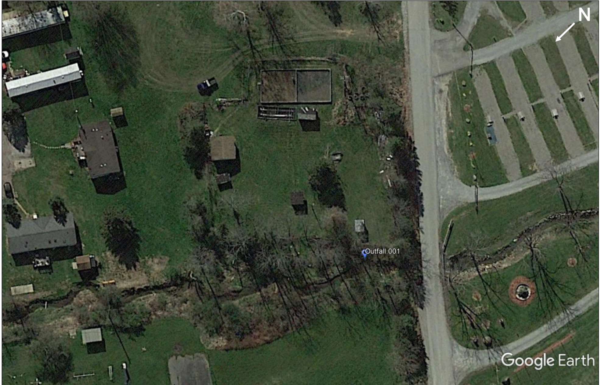
Aerial Image of STP and Outfall 001; Image Source and Date: Google Earth Pro, April 2016.
