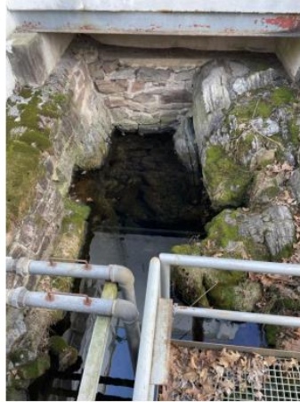
Photo by Shawn Lesitsky on 2/14/2023. Natural spring where non-contact cooling water is drafted from.
