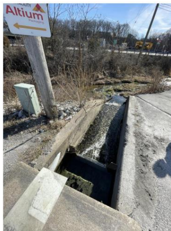
Photo by Shawn Lesitsky on 2/14/2023. Outfall 001 discharging non-contact cooling water and spring water into a UNT of Codorus Creek.
