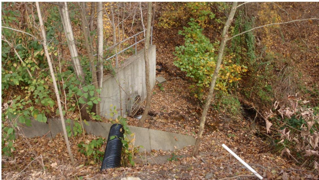
Figure 5: Structures at Fern Valley Outfalls 004 (background), 005, 006 and the Receiving Stream
