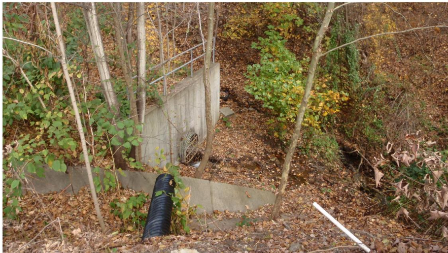
Figure 1: Structures at Fern Valley Outfalls 004 (background), 005, 006 and the Receiving Stream
