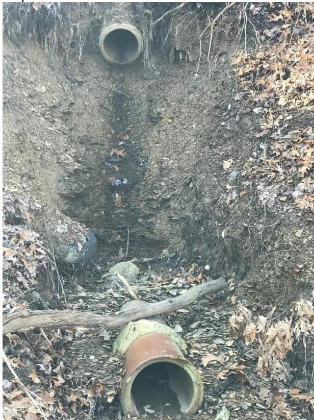
During high precipitation events, stormwater that is to be conveyed along the eastern side of Pond C will discharge to the Pond due to grading issues in this area. The stormwater pipe appears to come from Walter Panek Park. The pipe needs repaired, and the grading needs restored to properly convey the stormwater from this pipe away from Pond C.
