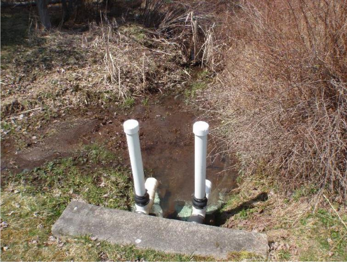
Figure 2. Outfall 001 structure showing the two discharge pipes
