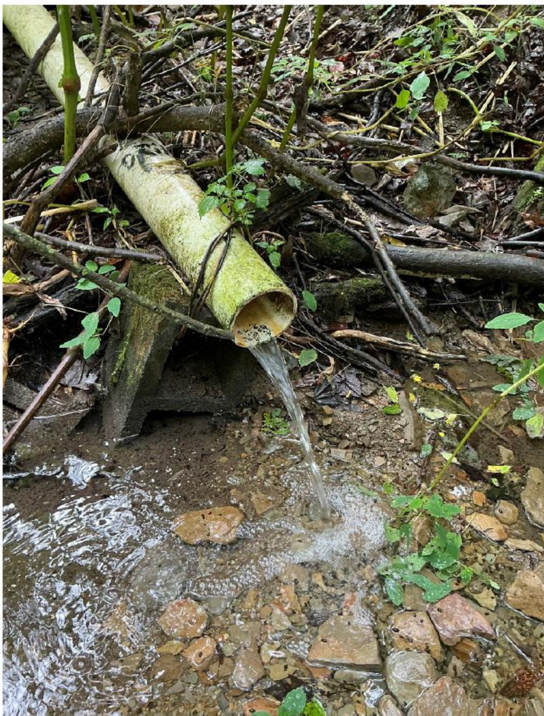
Figure 4. Knobvue Estates MHP Sewage Treatment Facility discharge outfall.
