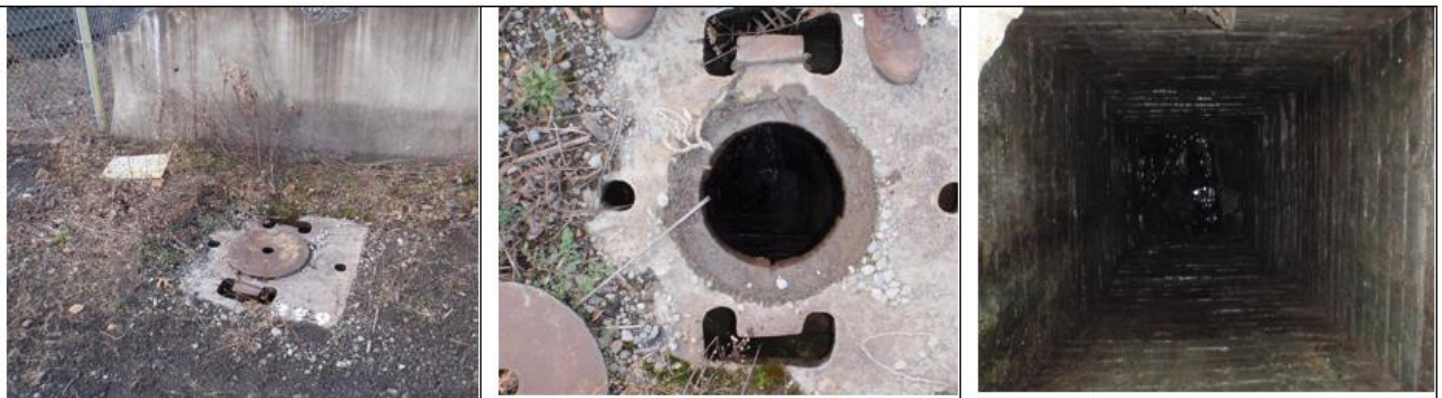
Figure 7: Pictures of the Manhole Sampling Point of JRS IMP 399
