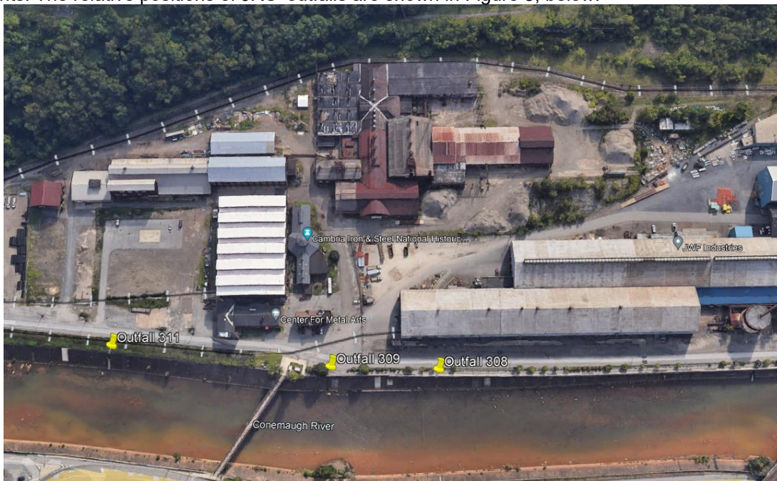
Figure 8: Annotated Satellite Image with Yellow Pins at Outfalls 308, 309 and 311
