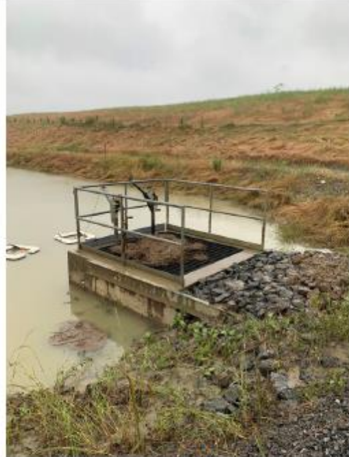
Photo #4 Partially Clogged Outfall Grate Photo Taken By: Brandon Bettinger on 6/11/2021
