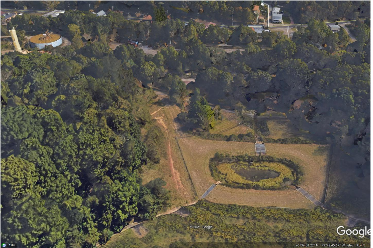
Figure 4: Cheswick Ash Disposal Site Sedimentation Pond and MMDP
