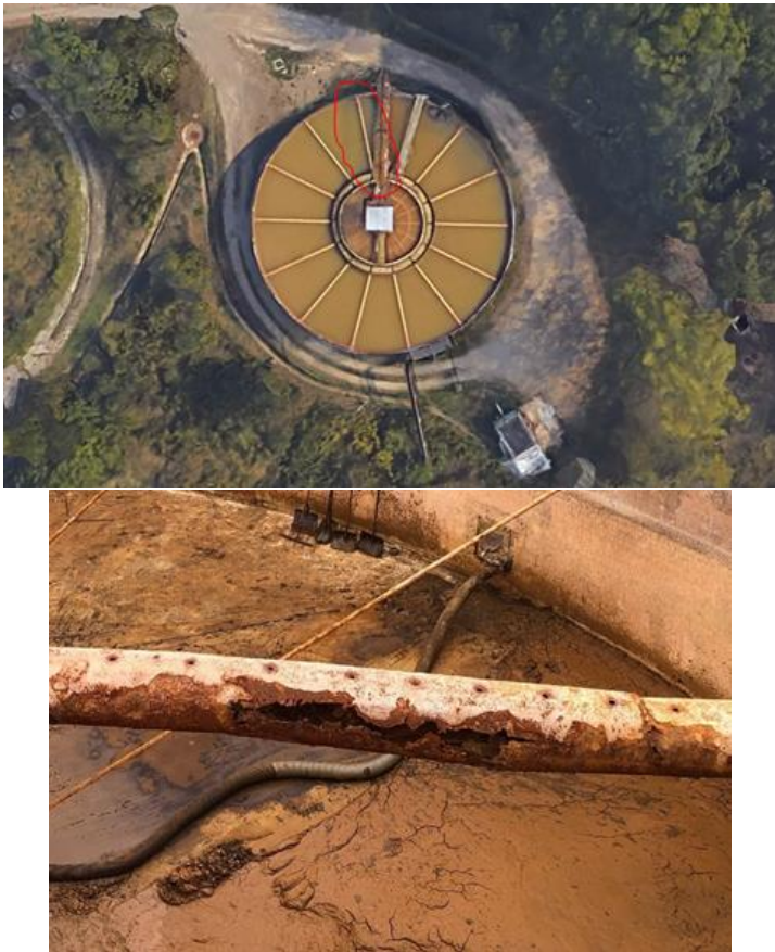
Figure 1: MMDP Clarifier highlighting the location of the faulted radial pipe and an image of the fault.
