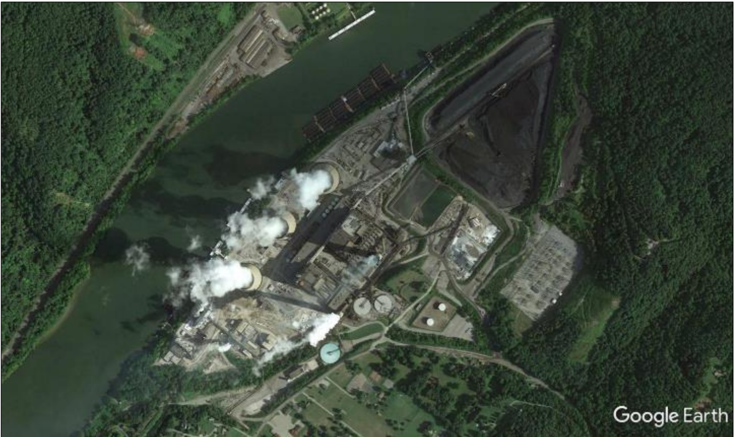
Pre-shutdown. Image Source and Date: Google Earth Pro, August 21, 2015.
