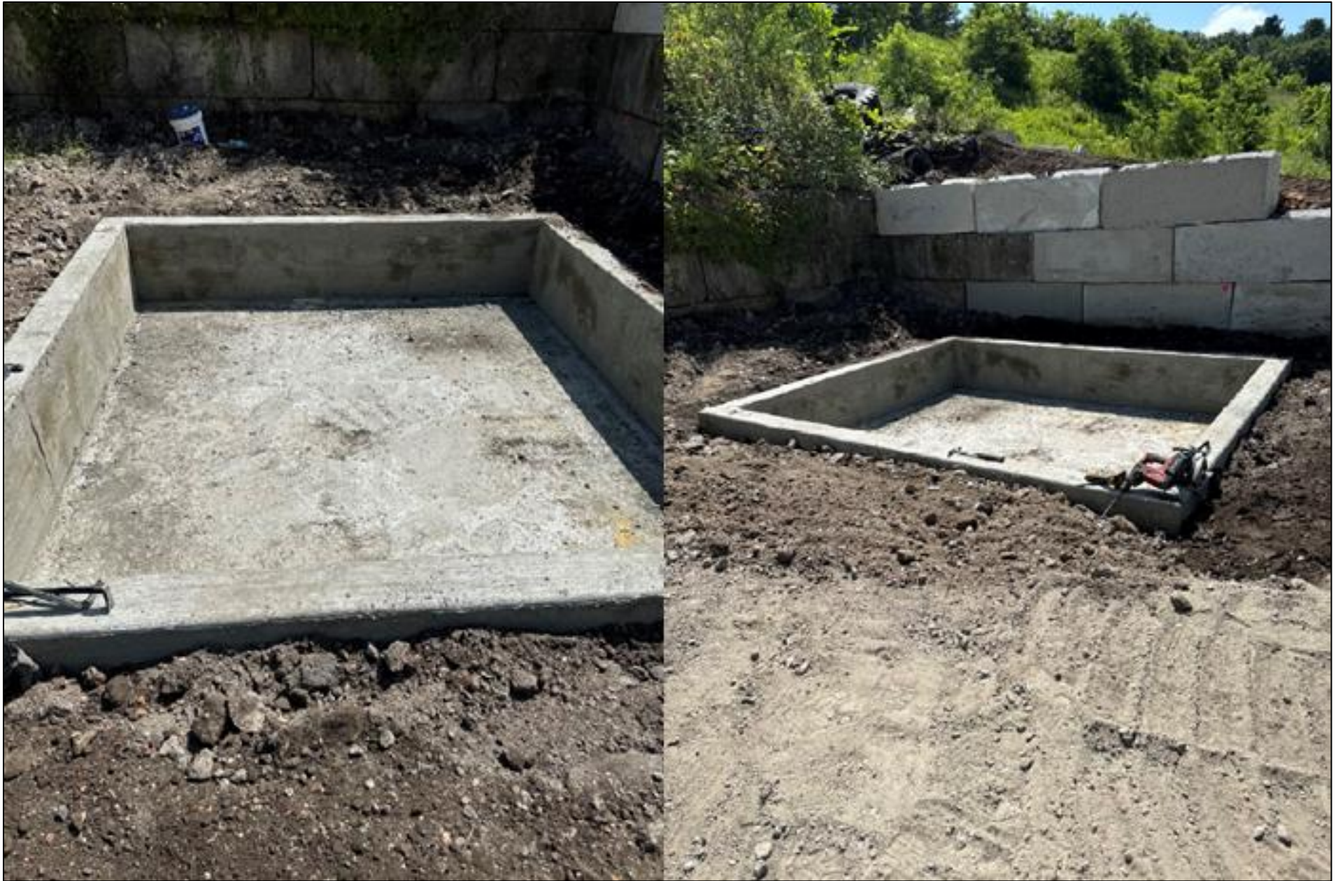
Figure 3. Newly constructed concrete truck barrel washout pit
