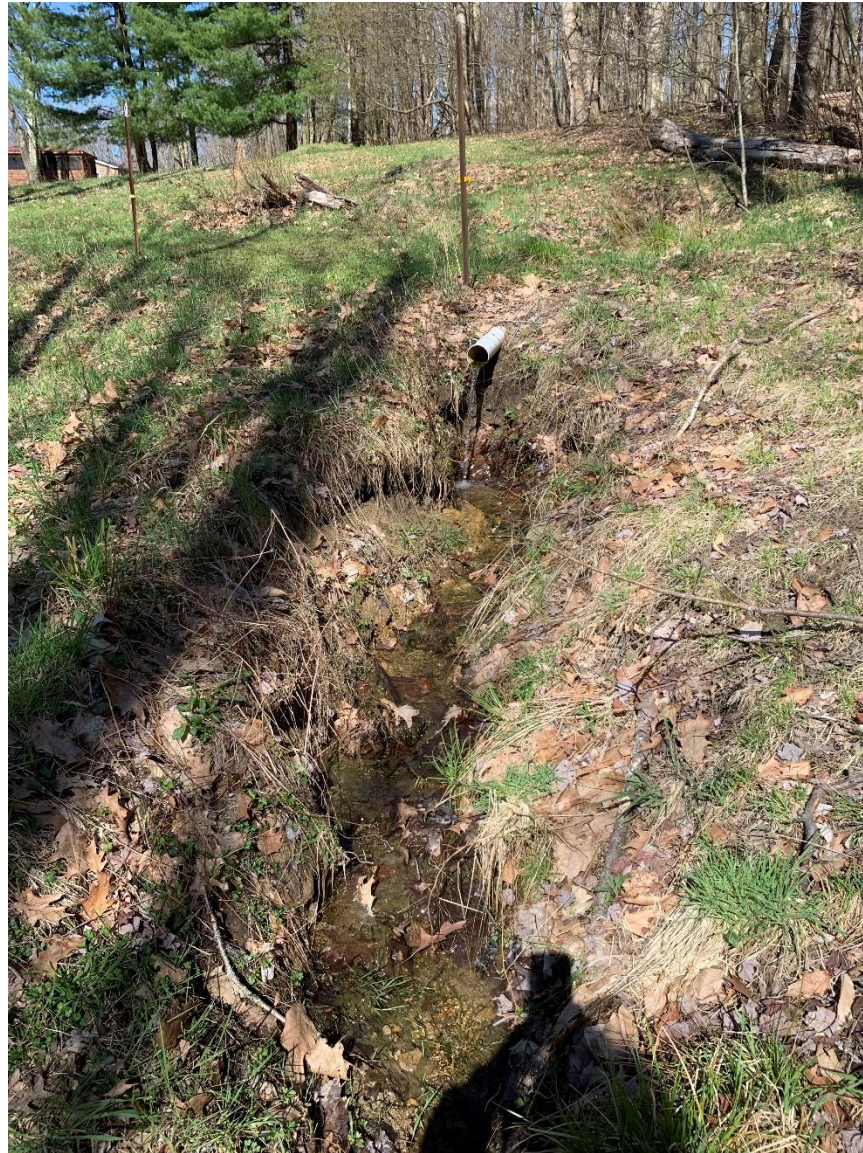
Photo 2: Spring fed drainage to pond. This is the area of the proposed outfall.
