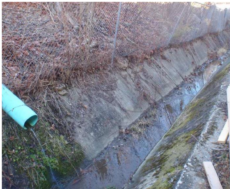
Figure 3: Drainage Culvert Running Along the Northwestern Perimeter of JWF's ETC Facility
