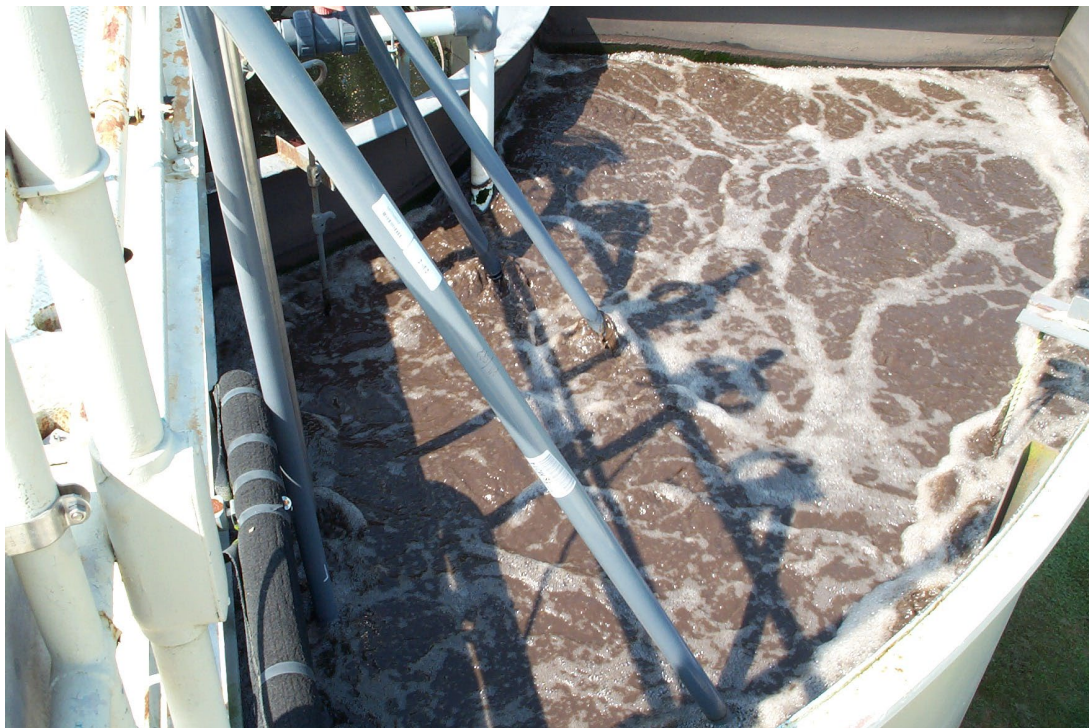
Figure F-6: Five Probes inserted at angle into Contact Tank 1
