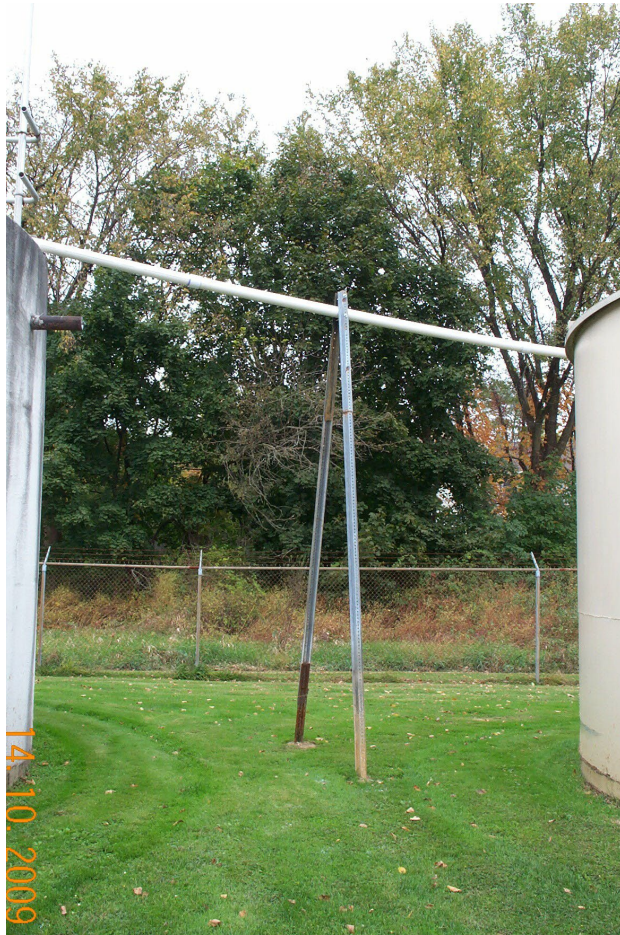
Figure 35: View of Temporary Raw Line & Support
