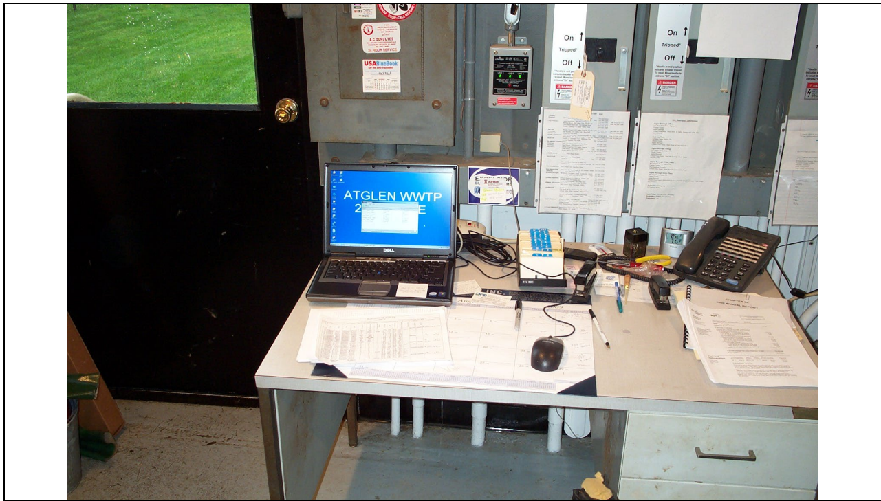
Figure F-7: Notebook Computer installed in Control Room and connected to SC-1000 Computer
