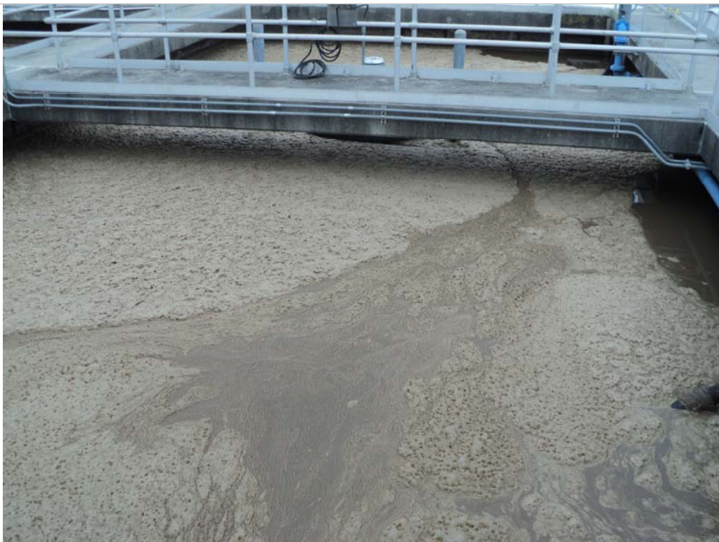
Figure 8: Foam buildup in Staged Aerobic Reactor Tank
