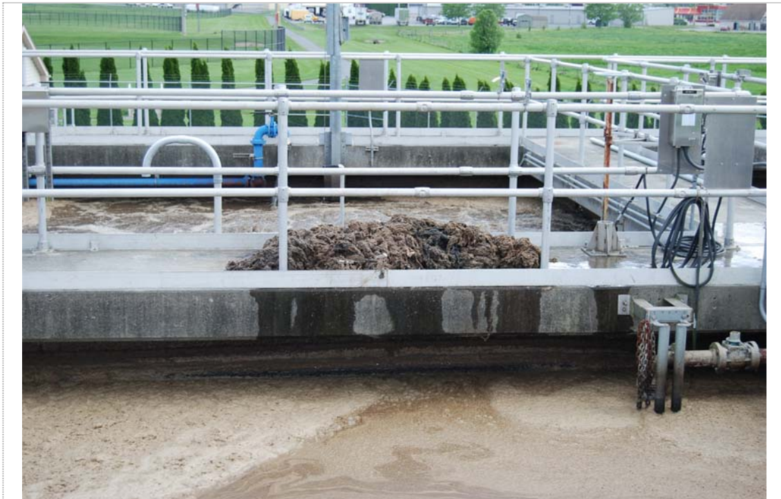
Figure 1: Large mound of rags and detritus removed from SAR
