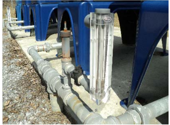
Photo 10: Aeration Rotometer & Relief Valve
