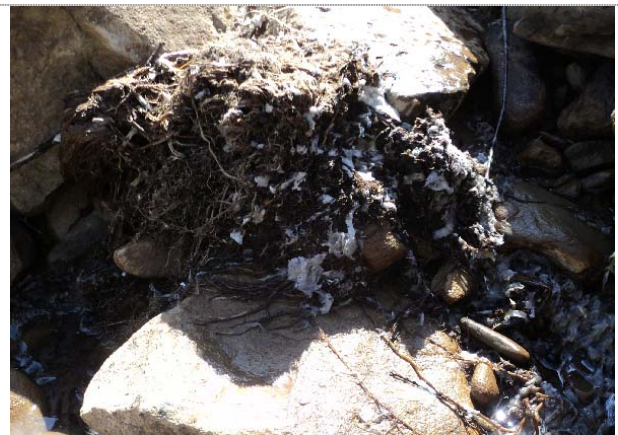
Photo 18: Detritus visible below outfall
