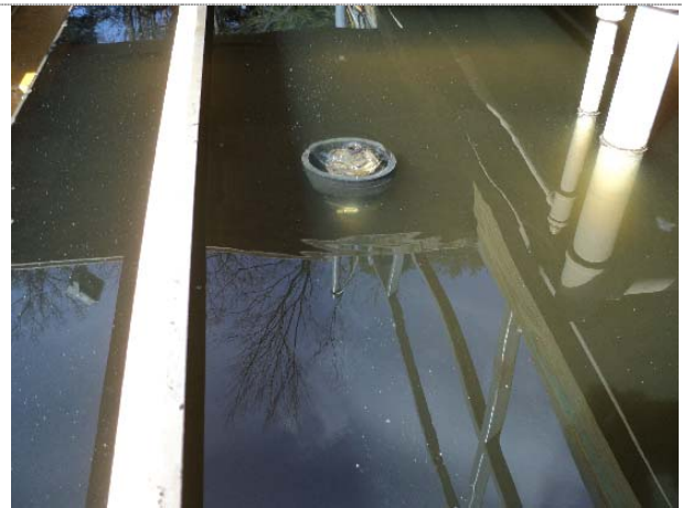
Photo 16: Adjusted scupper / clarifier quieted
