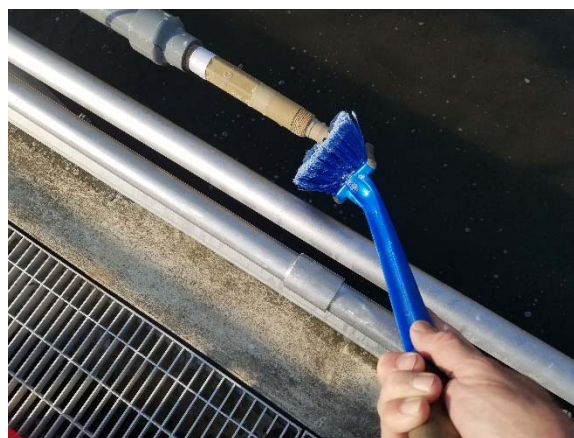
Photo 3: Clean probes regularly on a schedule
