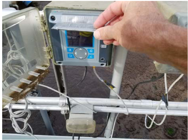
Completed sun shade
