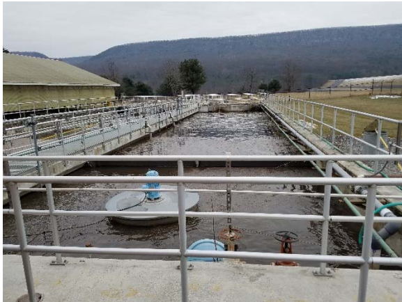
Photo 6: Secondary Treatment Train
