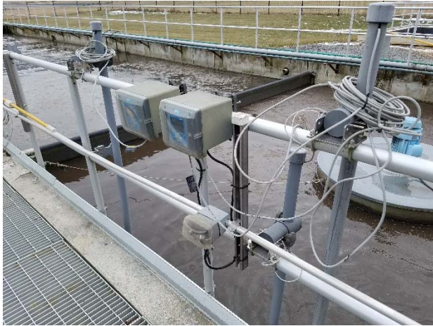
Existing Probe and Controller Installations
