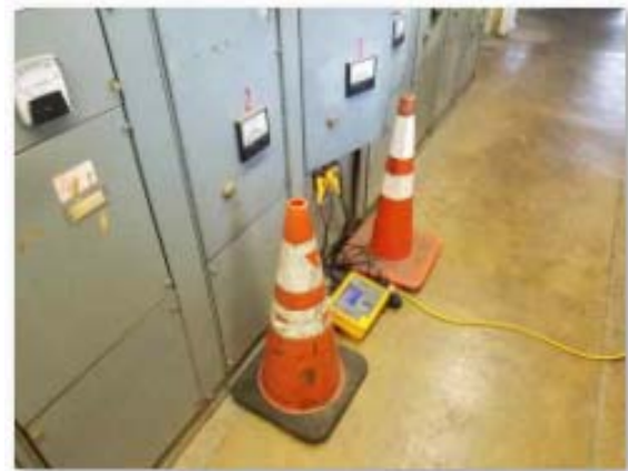
Power Logger for Centrifugal Blower Motor
