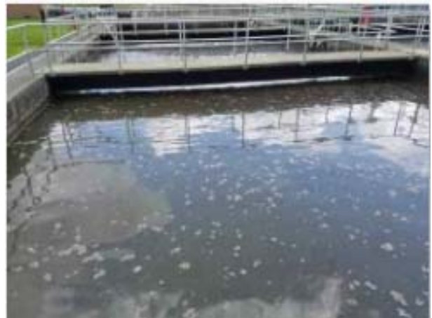
Aeration Tank during Anoxic Settling Period
