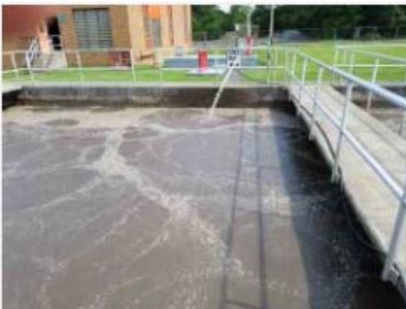
Biomass Under Aeration
