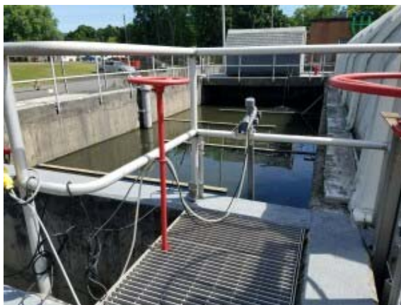
Ammonium & Nitrate Probes at Effluent
