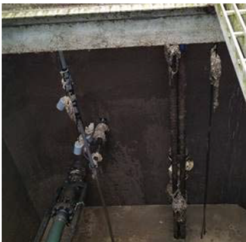
Photo of rags and debris: The weight of these masses, in the turbulence of stirred mixed liquor, will damage electrical cables and cause ground faults.
