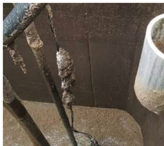
Photo of rags and debris: The weight of these masses, in the turbulence of stirred mixed liquor, will damage electrical cables and cause ground faults.
