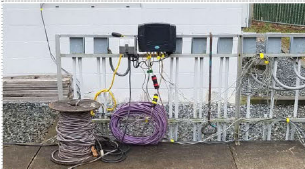
Probe controller set up by DEP
