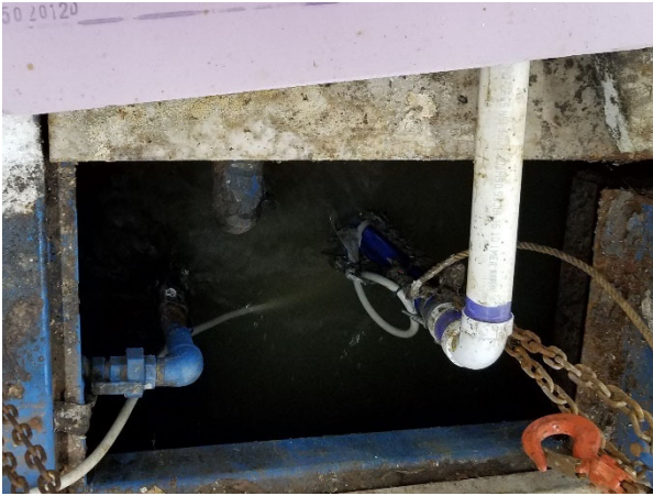
Influent splitter bypass pump
