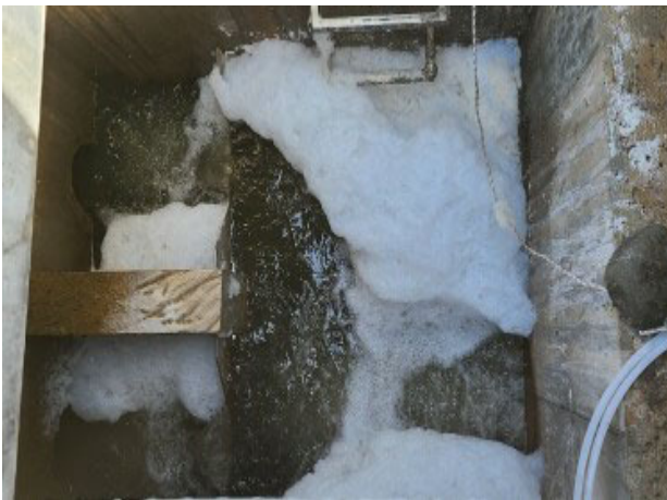
Foaming in Filter Influent Splitter Box
