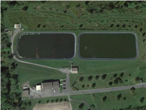
Aerial Overview of Treatment Facility
