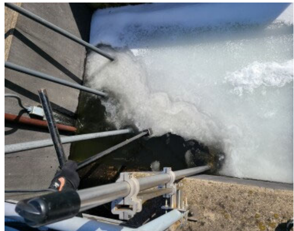
Surface ice forming around effluent probes
