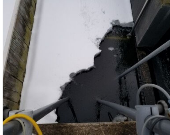
Monitoring probes near effluent pit
