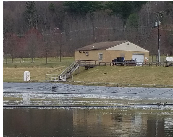
View of Control Building & Headworks
