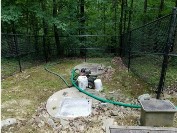
Disinfection & Sulfonation Wet Wells
