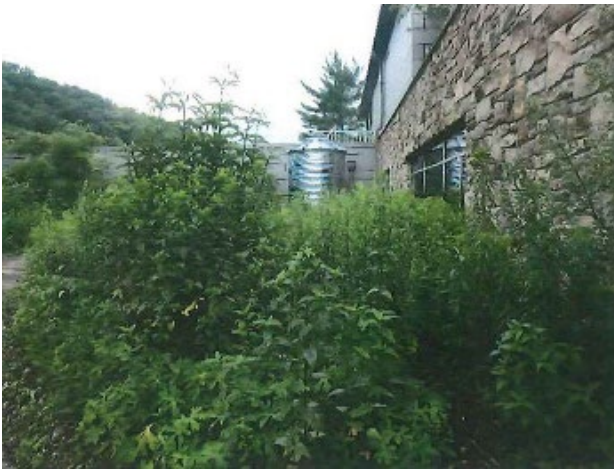
Rainwater Collection Zone
