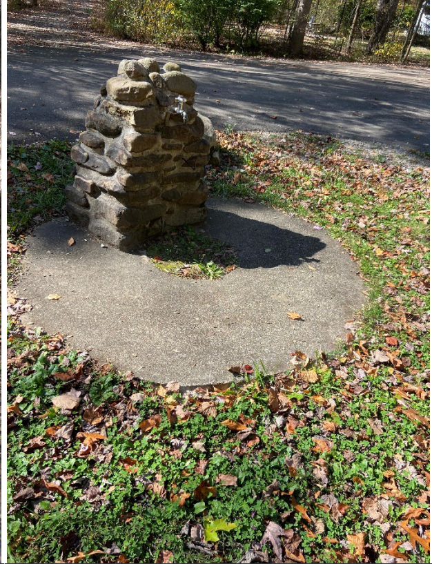
Potable water station with drainage pit below ground. Smoke was seen around concrete base.
