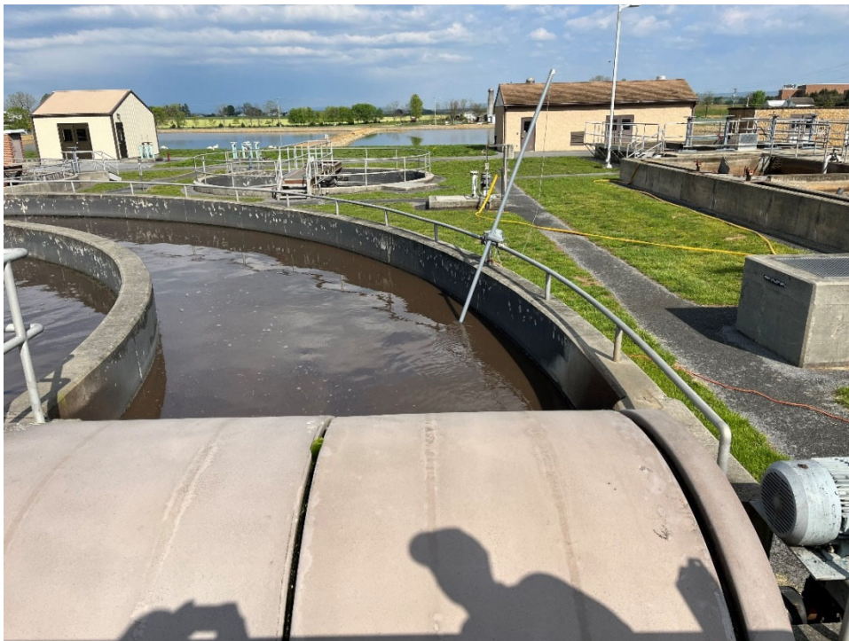
View of dissolved O 2 probe assembly in outer ring of Orbal, near brush rotor.
