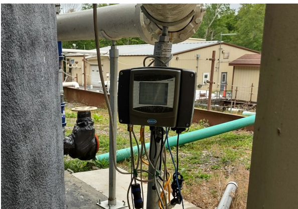
Probe Controller & Data Processor
