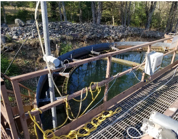
Ammonium Probe with Air-Blast Cleaning
