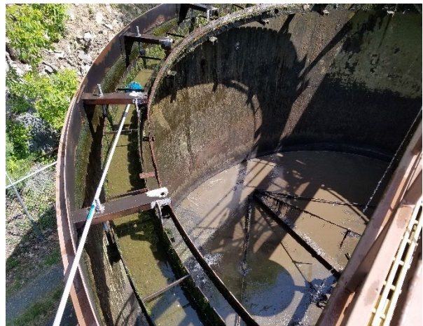
Cleaning Weirs while Clarifier emptied for air-lift pump modifications
