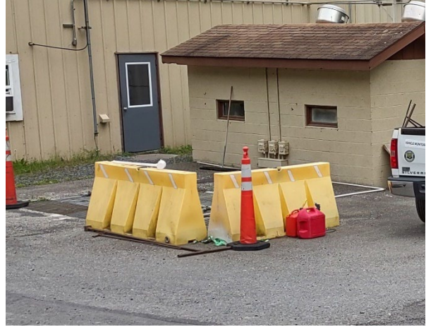
Sulfite Contact Tank in Ground
