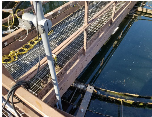
Nitrate Probe between tank wall and weir
