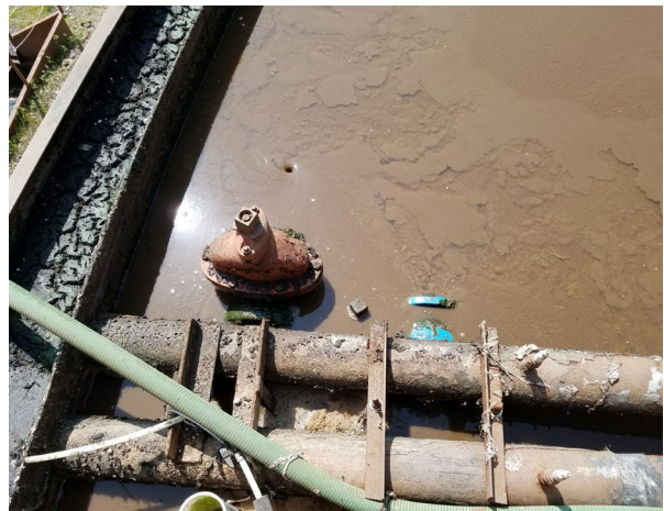
Siphoning of mixed liquor during OFF cycle
