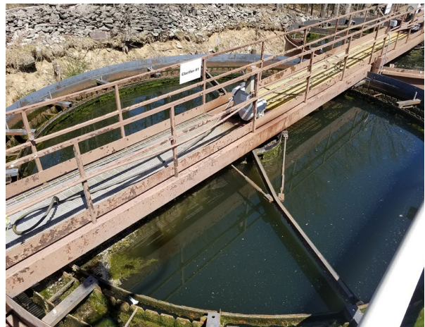
View of Secondary Clarifiers
