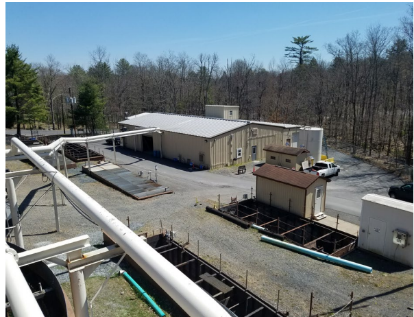
Five Equalization Tanks, Headworks, & Control / Filter Building
