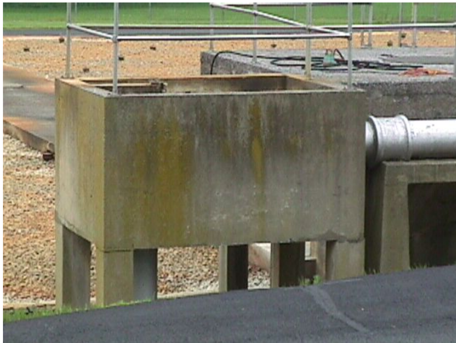
Figure 1.4 Dosing Chamber for Stationary Trickling Filters
