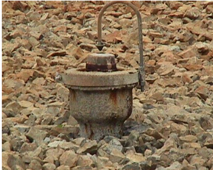
Figure 1.6 Spray Head for a Stationary Trickling Filter
