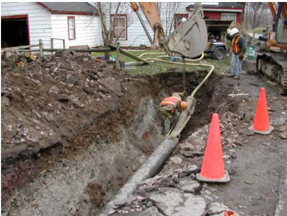
Bore and jack operation during construction
