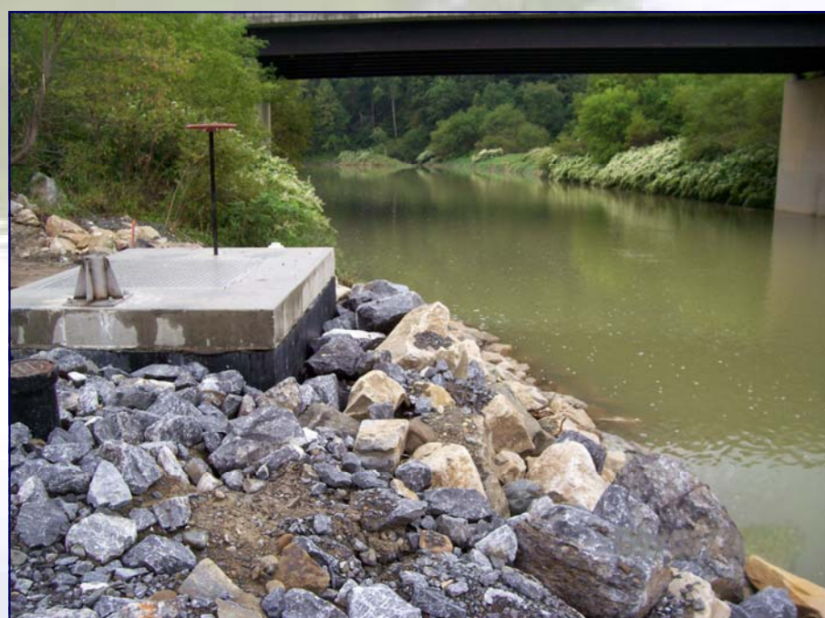
Finished River Intake Wetwell
