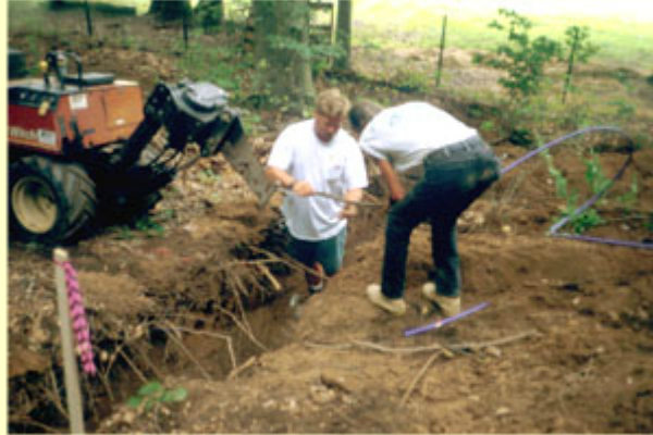
Header ditch for manifold
